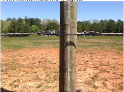
Figure 3 - Heliformed Suspension Units – used as intermediate attachments between dead ends for span lengths up to 2000 feet and line angles due to changes in elevation or direction up to 30
